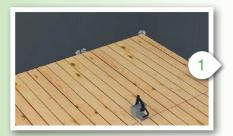
Put shower tray in the correct position and mark around the tray, to establish which section of the floor boards needs to be removed, the tray can be recessed.
