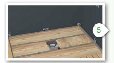
Once you are satisfied with the drainage, place plywood around the drain and fix in position.
